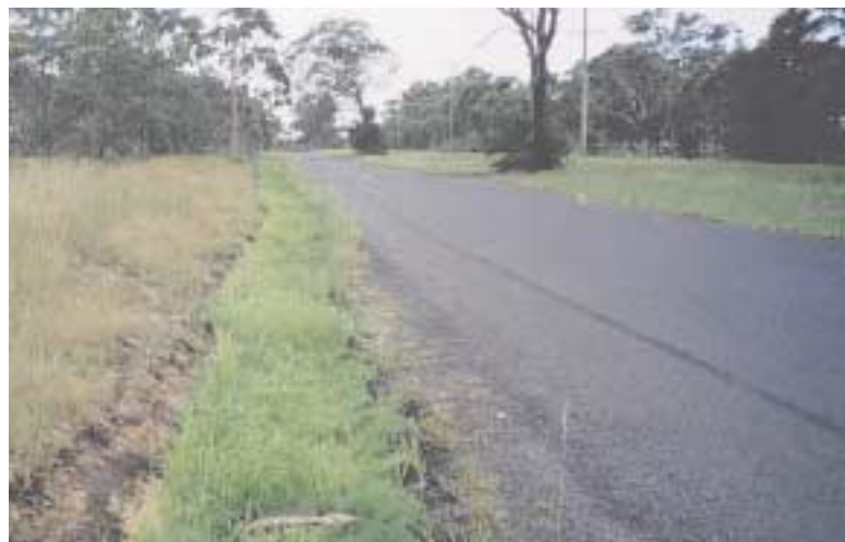
Eroded drainage line being reshaped ready for grassing at Chain Valley Bay. (And below) The same drain at Chain Valley Bay with established vegetation.
