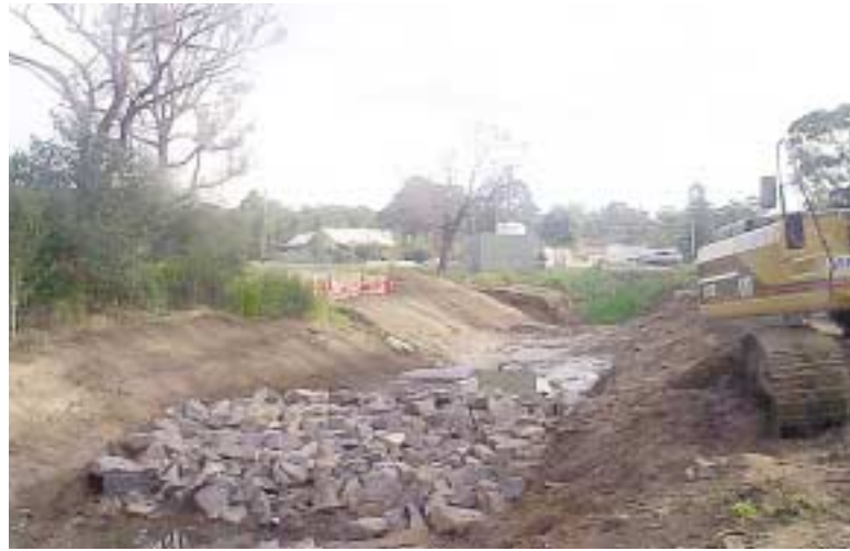
Wetland under construction, opposite Todd Street, Blackalls Park
