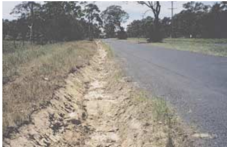
Eroded drainage line being reshaped ready for grassing at Chain Valley Bay. (And below) The same drain at Chain Valley Bay with established vegetation.
