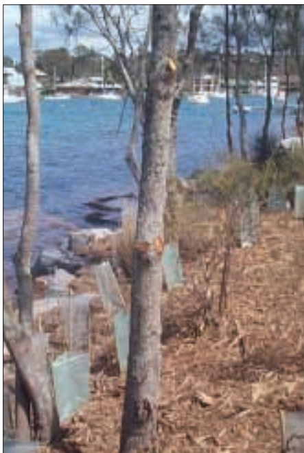
Balmoral Foreshore Reserve Stabilisation Works
