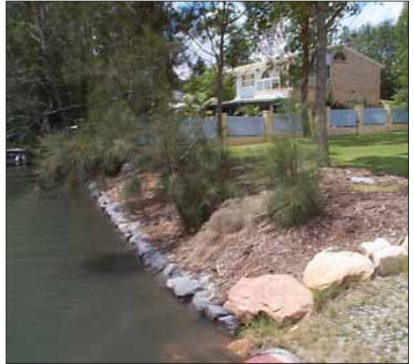
Creek bank stabilisation and riparian rehabilitation along LT Creek, Fennell Bay
