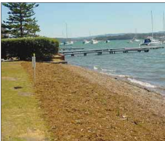
Foreshore stabilisation and beach reconstruction at Valentine Crescent, Valentine
