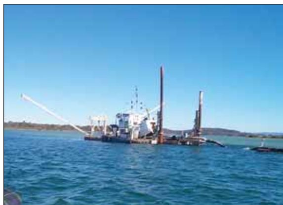
Maintenance dredging of Swansea entrance channel.
