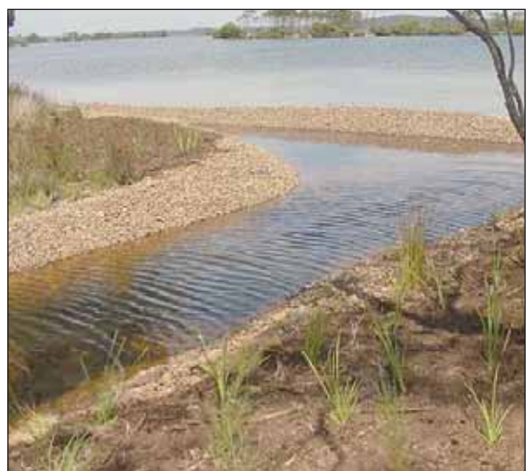
Drain outlet improvement works at Swansea Flats Reserve, Swansea.
