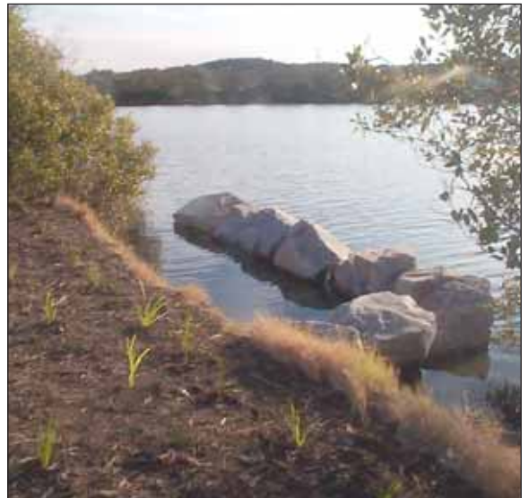
Erosion protection fillets at Creek Reserve Road, Boolaroo.
