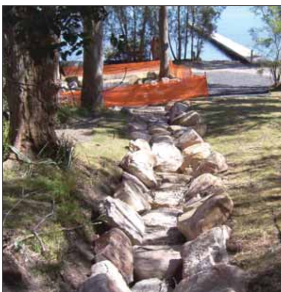
Drainage system improvements at Mulloway Road, Chain Valley Bay.
