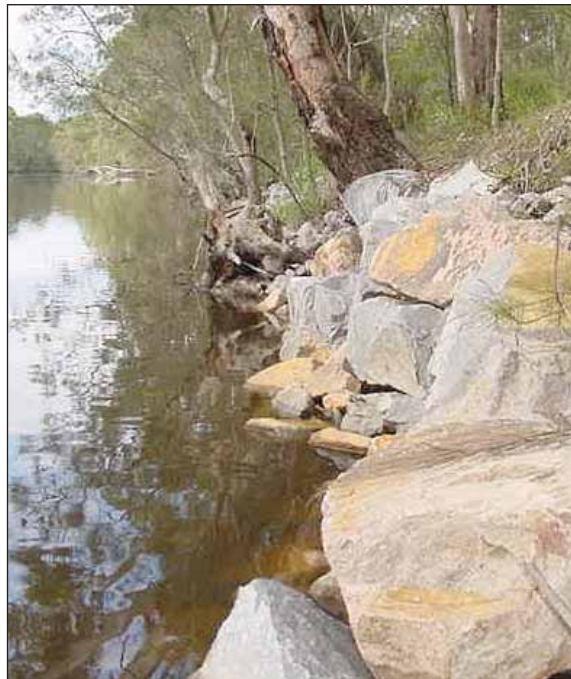
Creek bank stabilisation. Beauty Point Road, Dora Creek.
