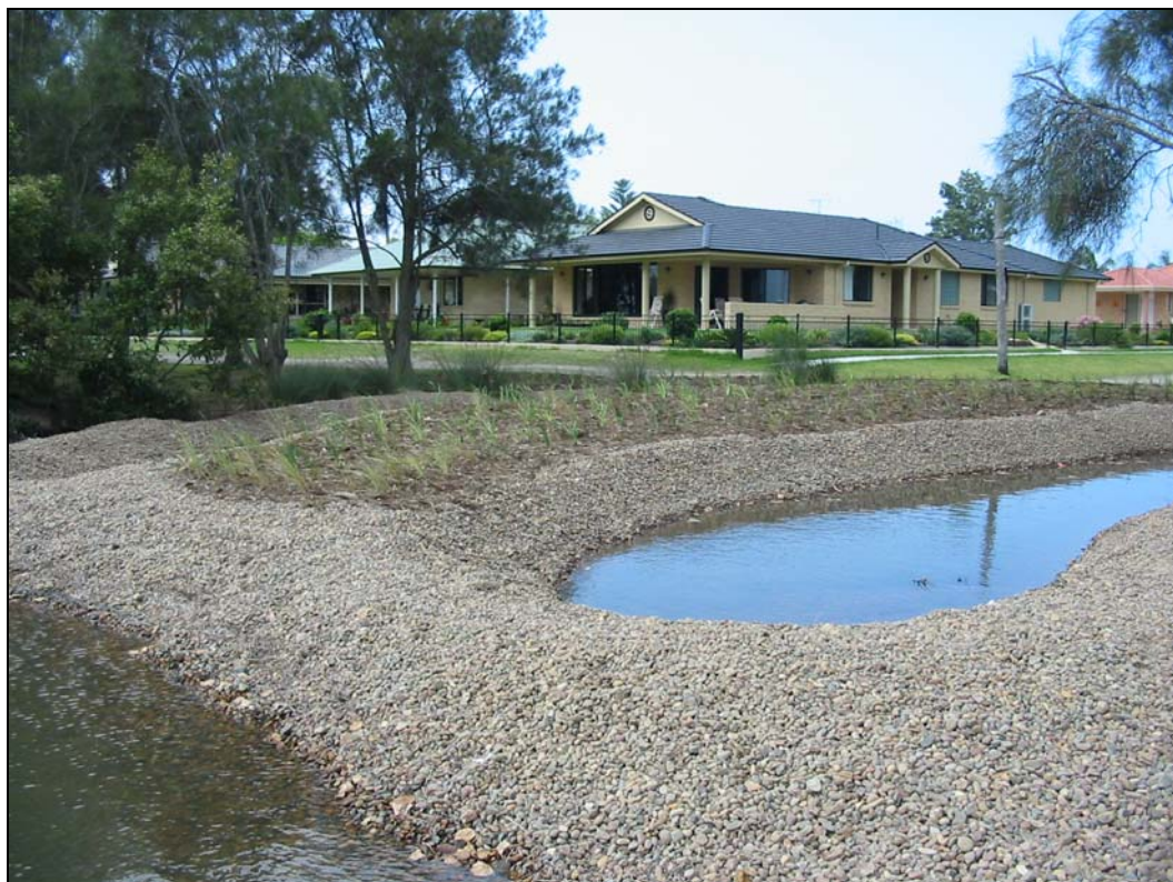
Figure 2.11 Stormwater Drain at Swansea Flats with cobblestone berm
