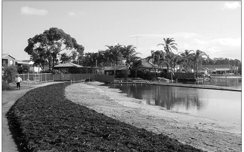
Organic sediment removal and beach re-creation during construction, Village Bay
