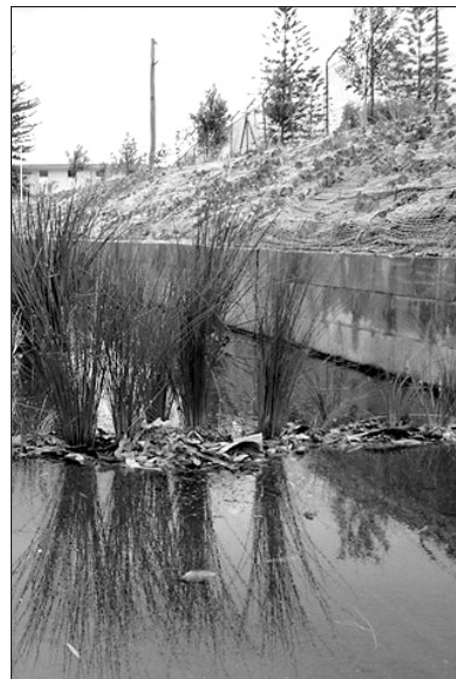
Concrete drainage channel improvements, Speers Point
