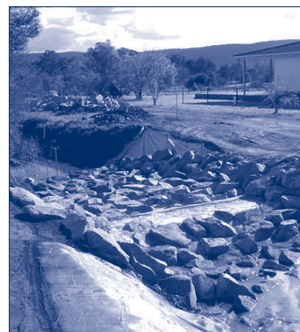
Works underway in West Wallsend
