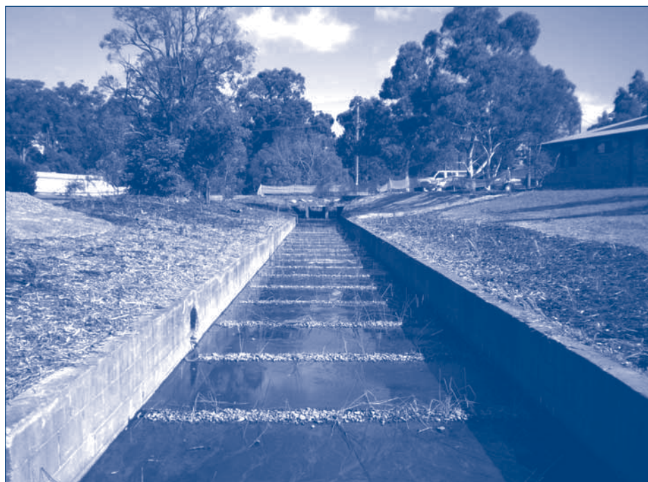
These vegetation filters, recently installed at Edgeworth, assist in improving water clarity.
