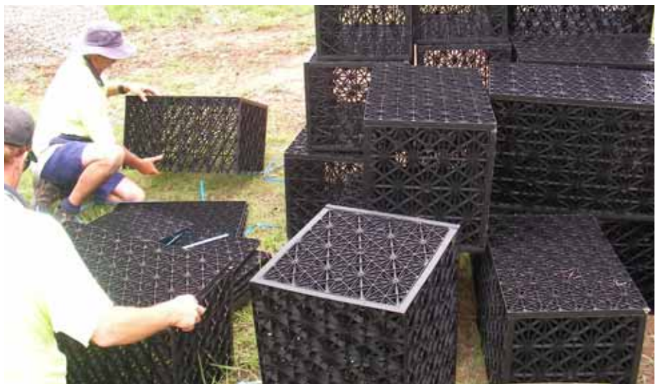
Workers preparing the Atlantis Cells
