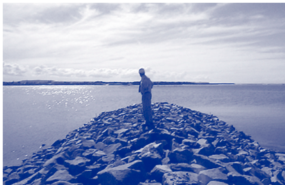
Richard Lack inspects the new rock groyne at Salts Bay
