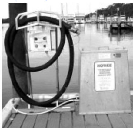
Example of a typical 'pump-out' (left) facility and 'slop-hopper'
