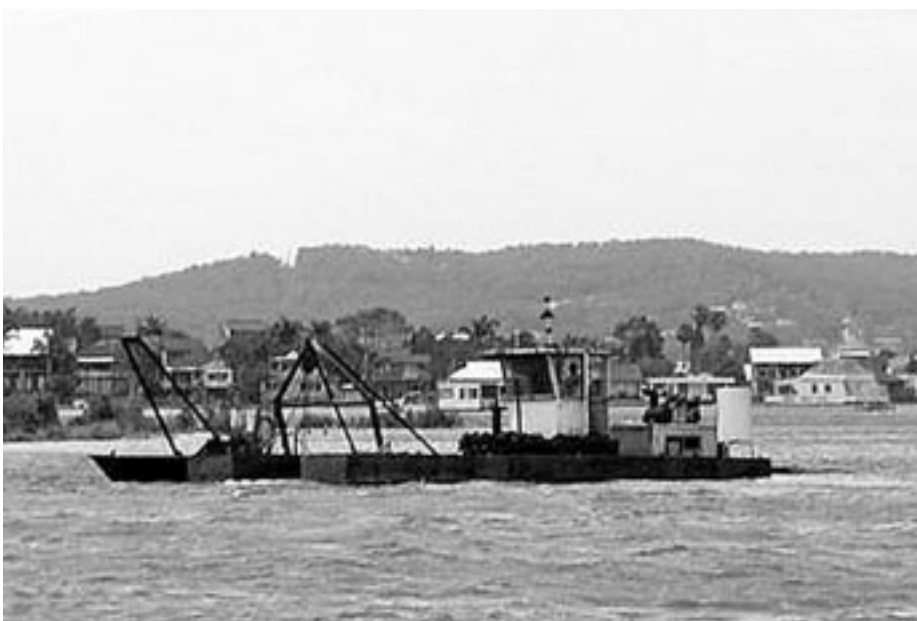
Maintenance dredging work in progress to improve boating access
