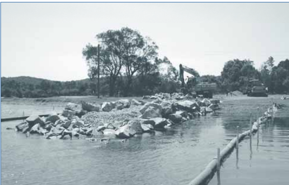
Cockle Creek groyne construction
