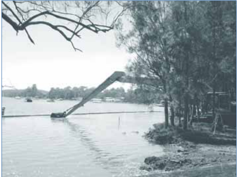
Bonnells Bay, nearshore organic sediment removal and foreshore rehabilitation works.
